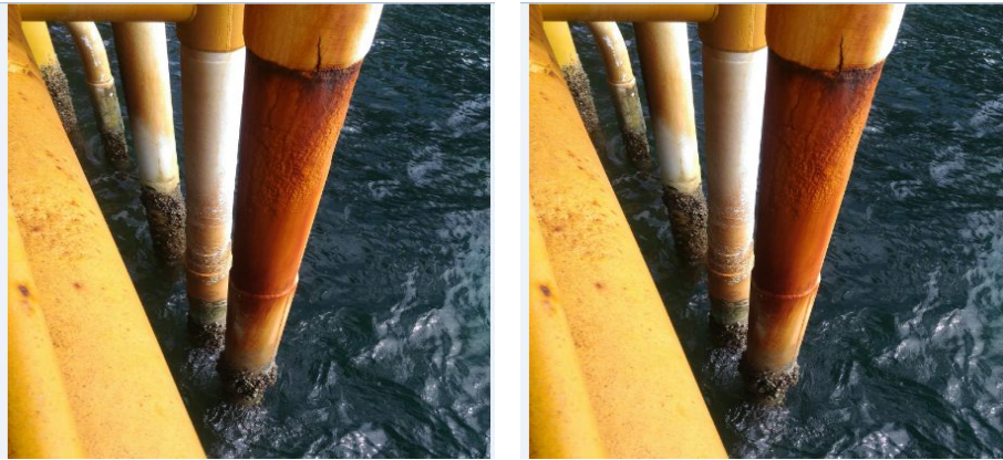
Error! Reference source not found. Riser pipa anjungan lepas pantai (Sumber koleksi foto Wakhid Yani K)
